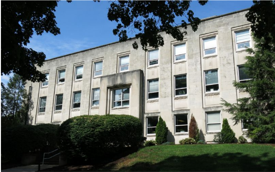
Kohr Administration Building – East facing façade:
