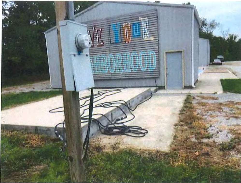
Photo 3. View of the building that was altered without permits August 2020. Photo by the Building Department.
